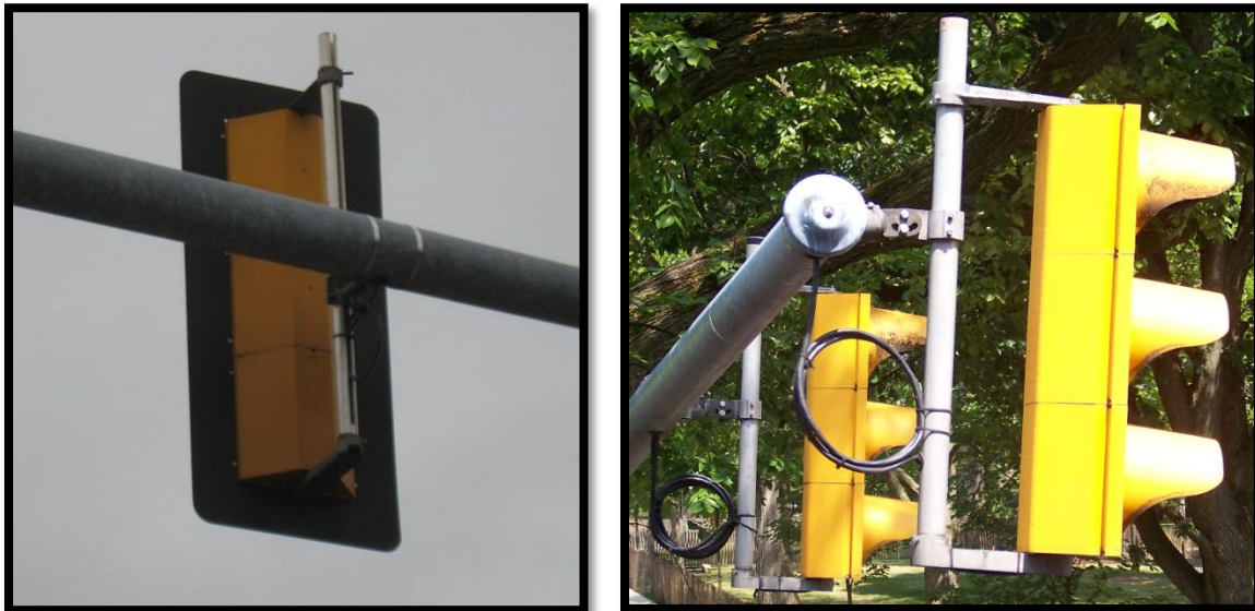
Exhibit 5-36 Traffic Signal Head Bracket System
