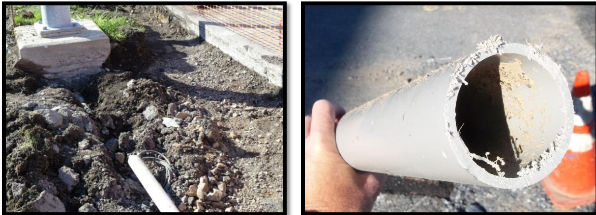
Exhibit 5-21 Conduit in Trench and Sample PVC
