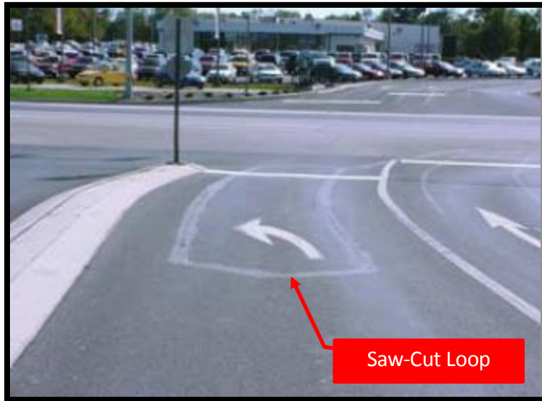
Exhibit 5-45 Inductive, Saw-Cut Loop Detector
